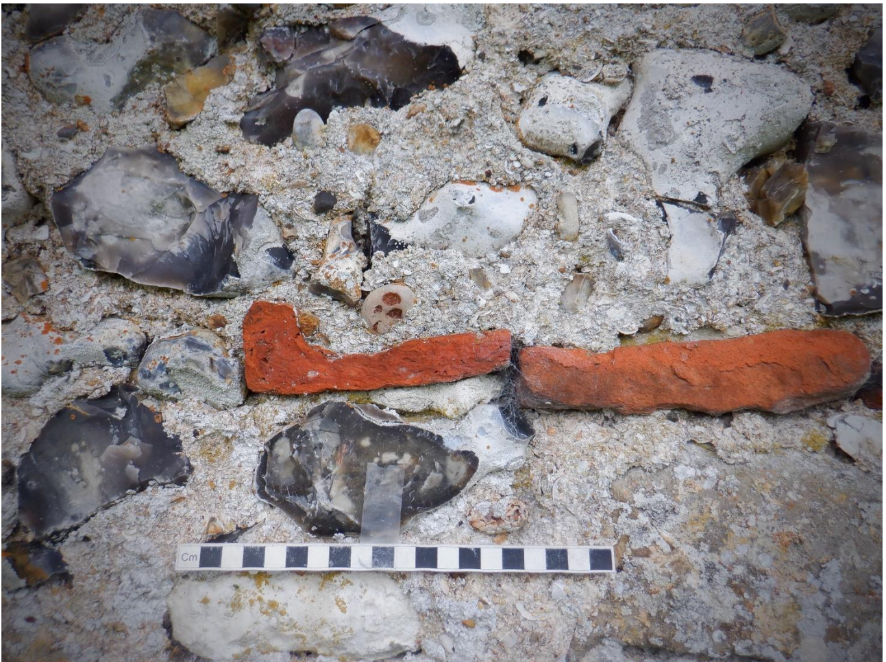
Plate 3: Fragments of Roman roof tiles- tegulae- used as levelling courses in the external walls of St Mary's Church. The amount of Roman building materials used strongly suggest the church is a Saxon rebuild of an earlier Roman building and worth comparing to the Church of St. Margaret of Antioch situated at Lower Halstow in a similar situation.
