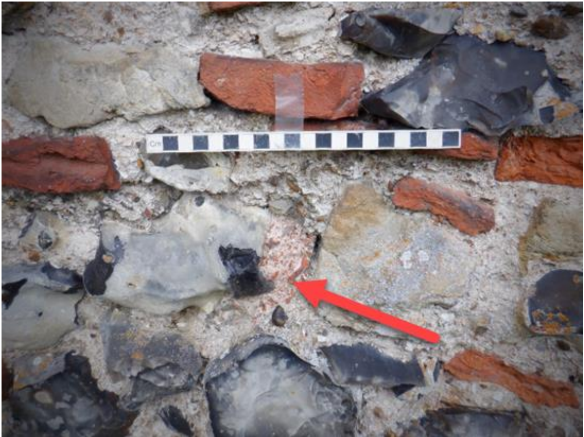
Plate 6: The east wall of Teynham church shows the reuse of Roman building material in the medieval structure including tegulae roof tiles and opus signinum flooring material (red arrow)
