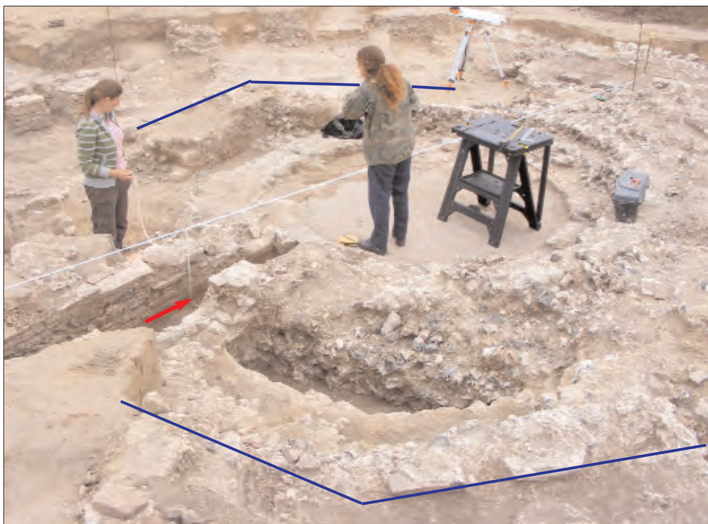
Fig. 52. Room 4 (above) situated in the centre of the building was built originally as a large octagonal plunge pool. The blue lines indicate the outside edge of this
