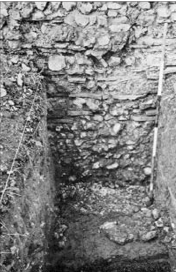
Fig. 22 The wall (left) is part of the structure of the cella ( Building A ). The build is unlikely to be of a Roman date, the layers of broken tiles, bricks and flints is in the same chaotic style as the early churches of St Martins in Canterbury, Lower Halstow, and Teynham most of which are reputed to have been built in the 7th-8th centuries.
