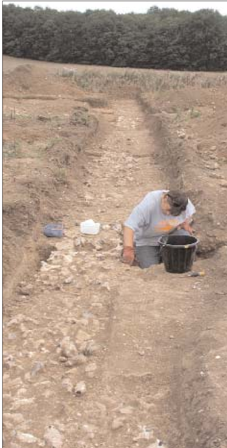
Fig. 67 A view of Trench 9 looking towards the north. The substantial stone mortared Roman perimeter wall can be seen running the entire length of Trench 9 before turning to the west.
