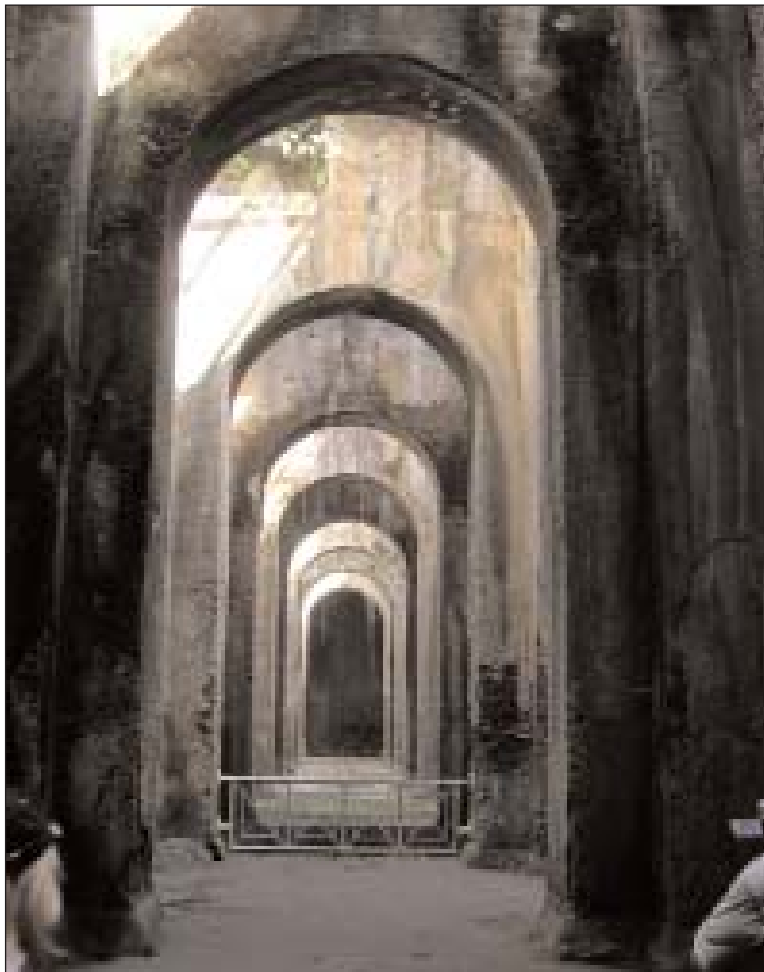
Fig. 25. The Piscina Mirabile at the Roman naval base of Misenum near Naples ( left ) utilises the use of the arch in five pillared aisles. Here the clerestory lighting illuminates the interior in exactly the same way as it would have done at Hog Brook. The photograph ( above ) of double brick lacing on the Roman lighthouse at Dover shows that this feature, also seen on the collapsed pier at Hog Brook was to bind together the courses of stone facing and core whilst the mortar was still soft. Another function was to level off the wall and keep the build horizontal.
